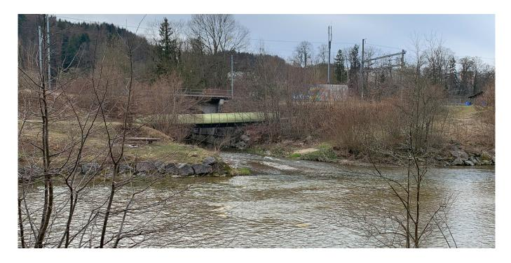
As part of the Swiss Federal Railways (SBB) project to increase its railway capacity between the cities of Zurich and Winterthur, we are planning a northward relocation of the confluence of the Kempt and Töss rivers so as to permit occasional floodwaters to flow under the new SBB crossing without flooding the planned Brütten Tunnel. We are also facilitating external physical model tests for testing optimizing our hydraulic engineering project.
